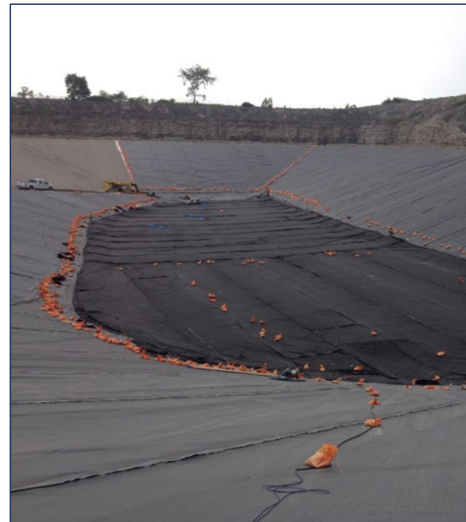
Above: Storage facility incorporates a high density polyethylene (HDPE) geomembrane liner underlain by a clay liner.
