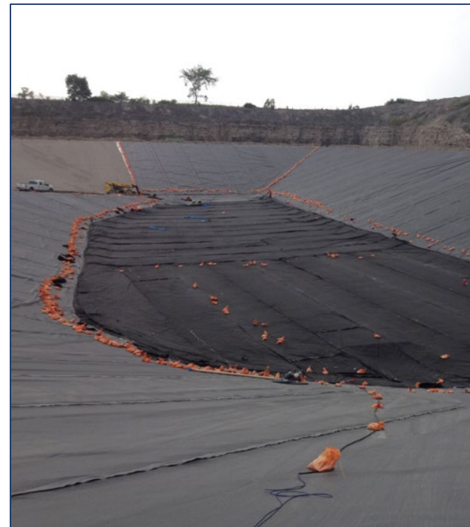
Above: Storage facility incorporates a high density polyethylene (HDPE) geomembrane liner underlain by a clay liner.
